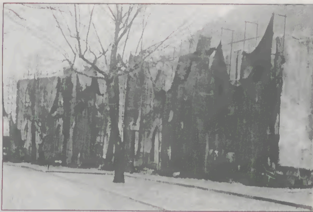
As ruínas do Hotel Ribeiro
