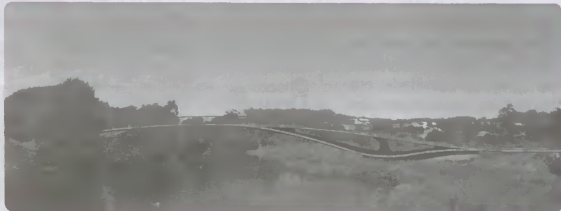
»»» Ponte pedonal do Rio Neiva
